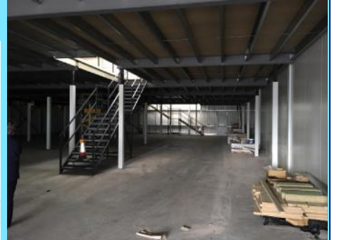
The mezzanine is now installed
